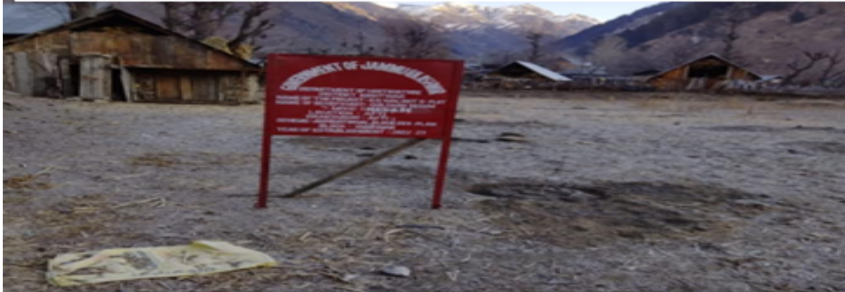
Warwan- Installation of sign board at D-Plot
